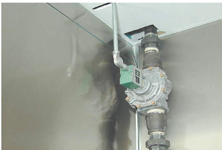
EXHIBIT 10.5 Solenoid for providing fuel shutoff.
