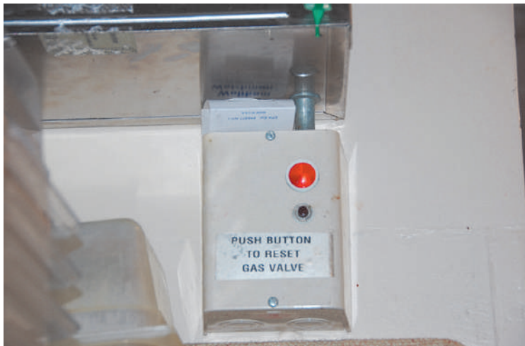
EXHIBIT 10.6 Manual reset for fuel and electric power.
