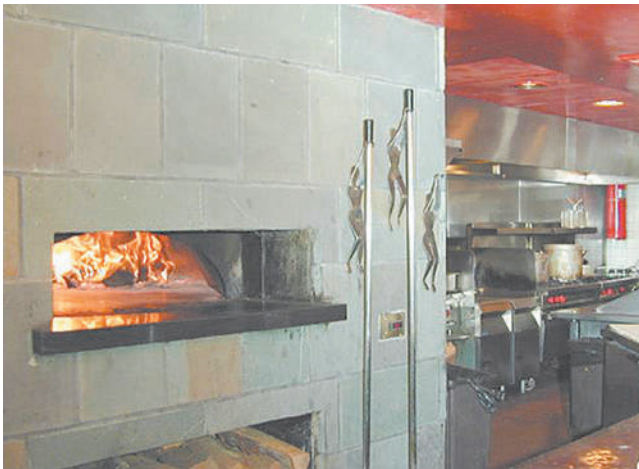
EXHIBIT 14.1 Example of a solid fuel cooking operation.
