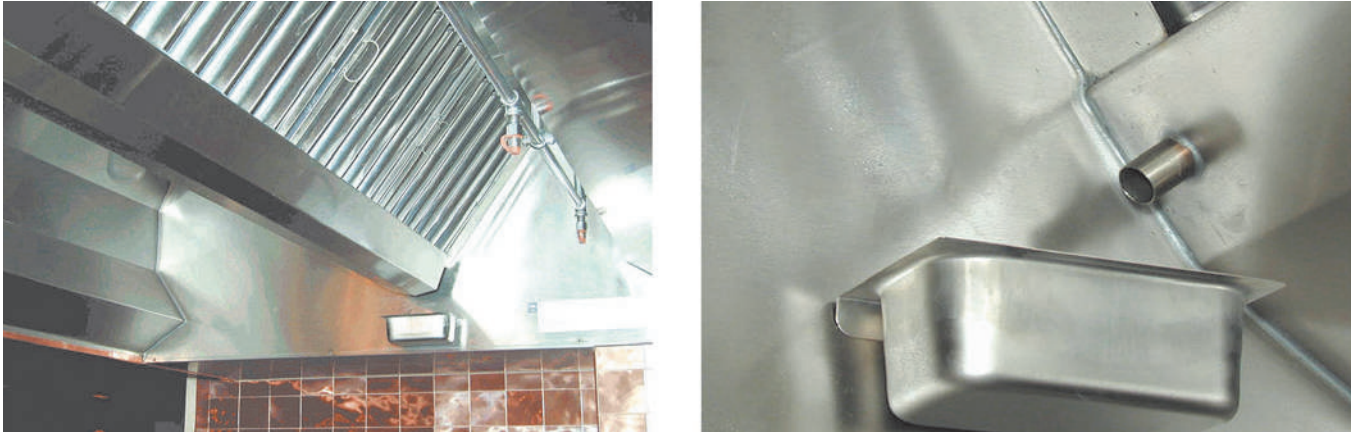
EXHIBIT 6.2 Examples of a grease drip tray.
