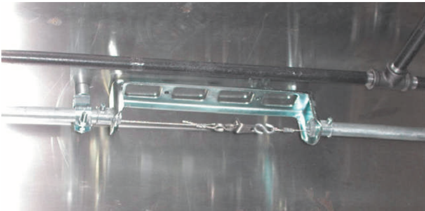
EXHIBIT 3.6 Example of a fusible link.
