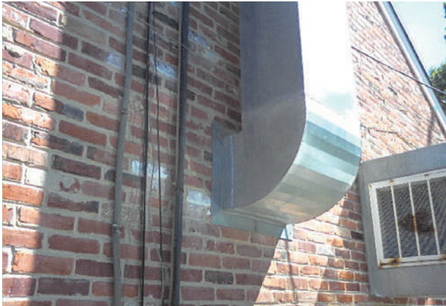
EXHIBIT 7.6 Example of a properly sealed penetration.
