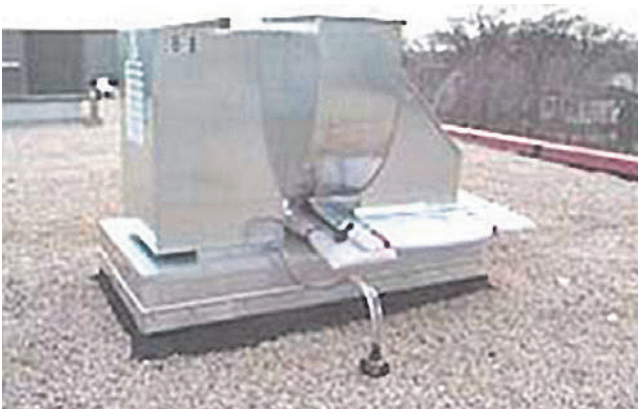
EXHIBIT 8.3 Example of a utility set exhaust fan.
