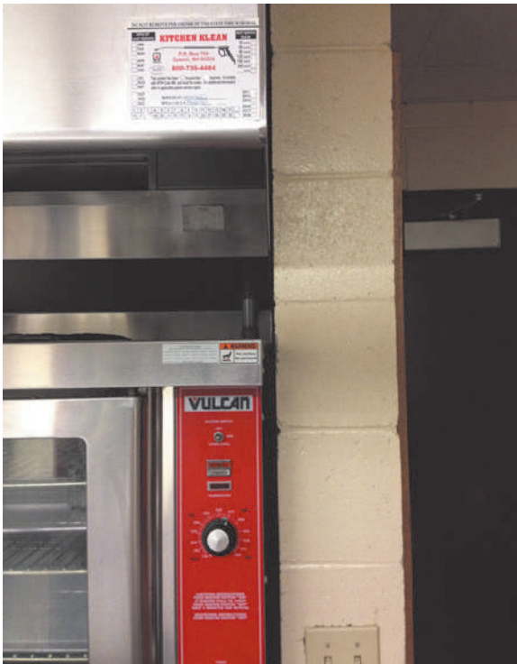
EXHIBIT 5.8 Hood over equipment with no overhang.
