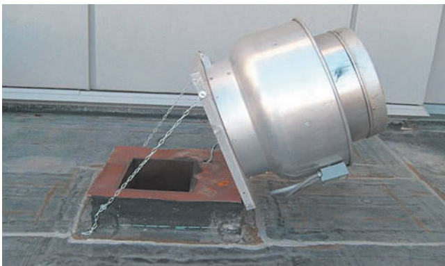
EXHIBIT 8.1 Hinged upblast fan. (Courtesy of the Delta Company, LLC)
