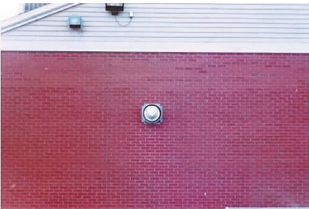
EXHIBIT 7.5 Wall termination provided with proper clearances.
