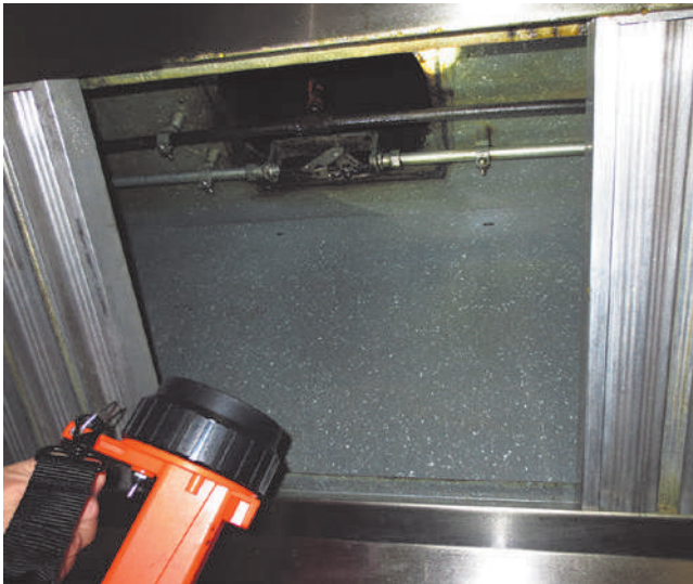
EXHIBIT 6.1 Example of a grease filter removed for inspection.
