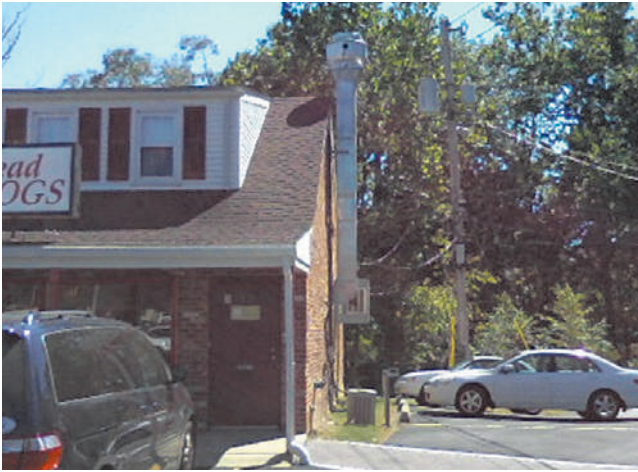
EXHIBIT 7.2 Exterior through-wall duct installation.
