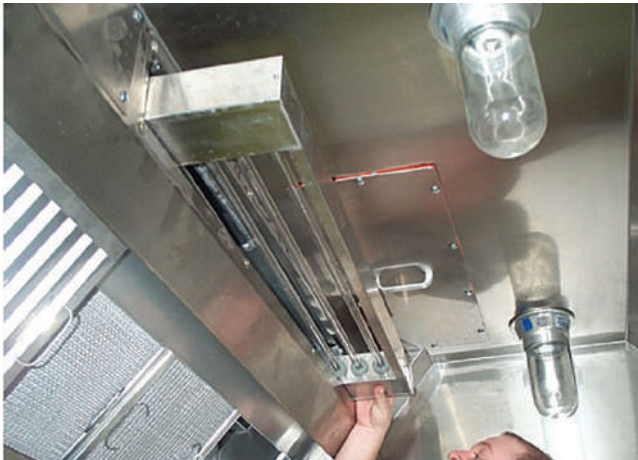
EXHIBIT 5.9 Ultraviolet hood. (Courtesy of Halton Company)
