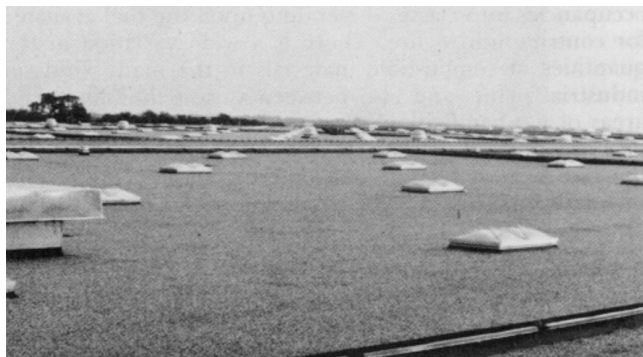
Figure A.1.1.1(b) View of Roof Vents on Building.
